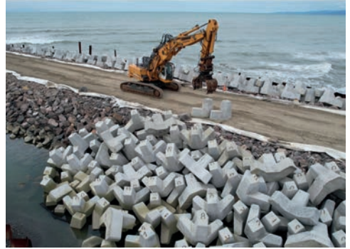
Hanbars being placed along seawall
