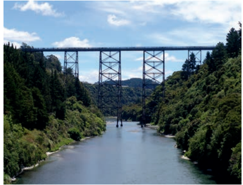
Mohaka Viaduct – photo courtesy of Wairoa District Council.
